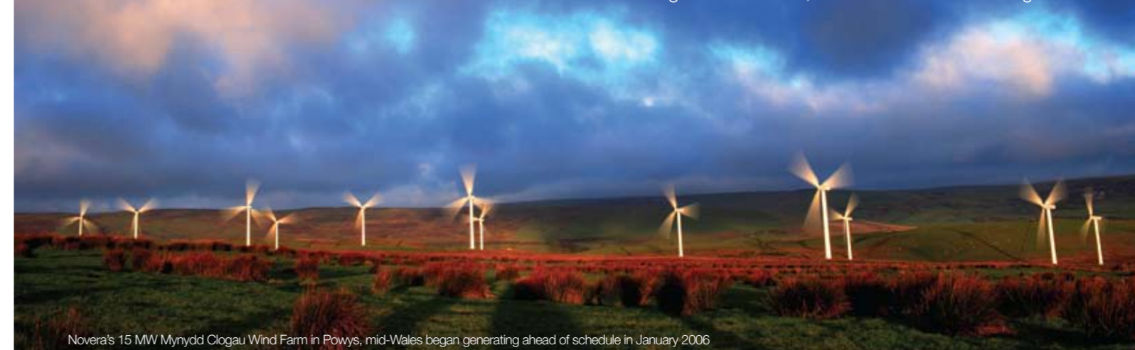
Novera's 15 MW Mynydd Clogau Wind Farm in Powys, mid-Wales began generating ahead of schedule in January 2006
